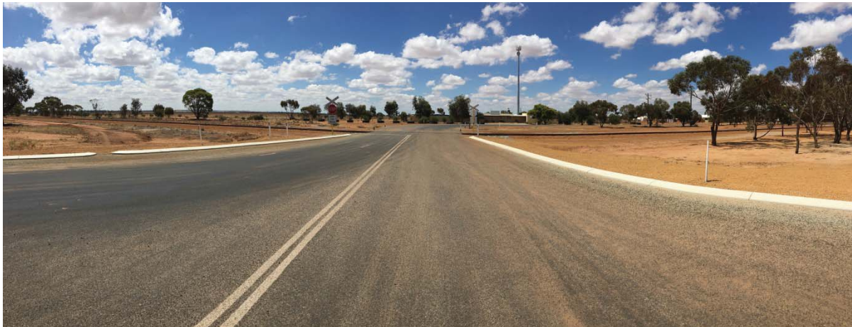
Above: North view of Railway crossing.
