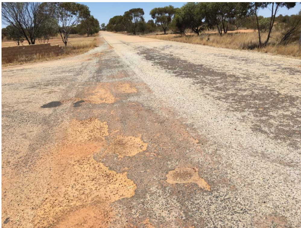
Above: Williams Drive / Earl Drive Intersection
